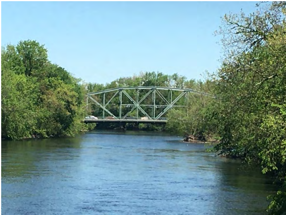
Straight Street Bridge
