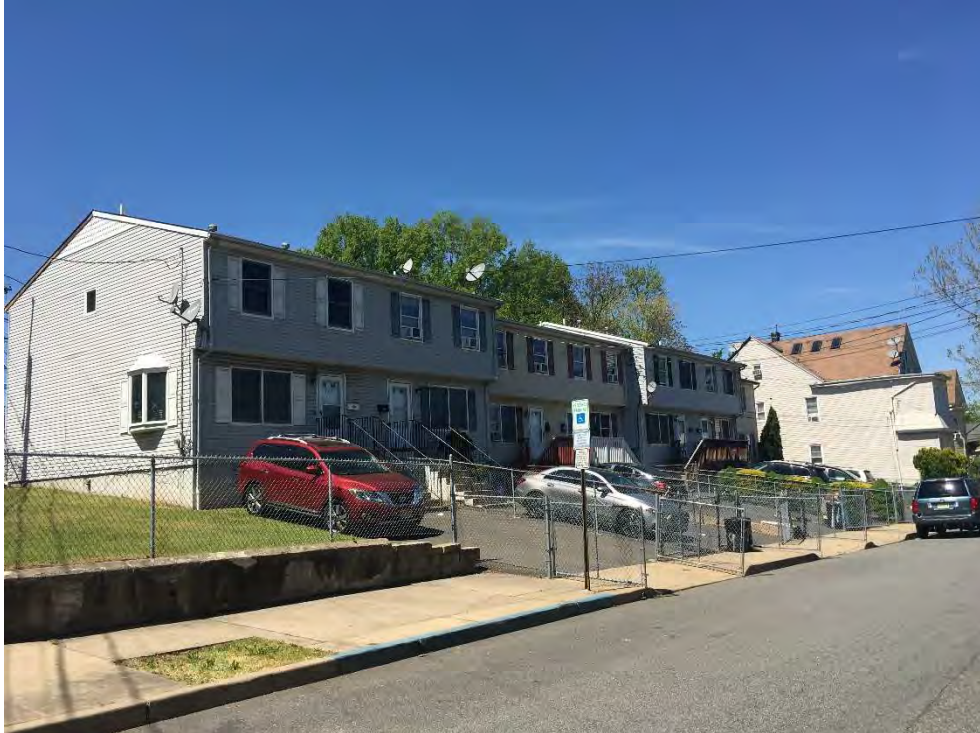
Attached homes on N. 1st St.
