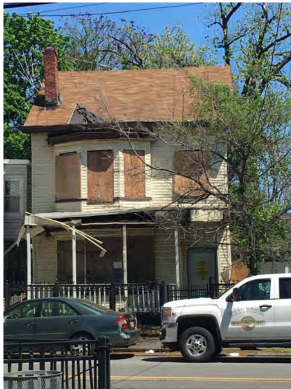
Abandoned home adjacent to Cobb Park on E. Main St.
