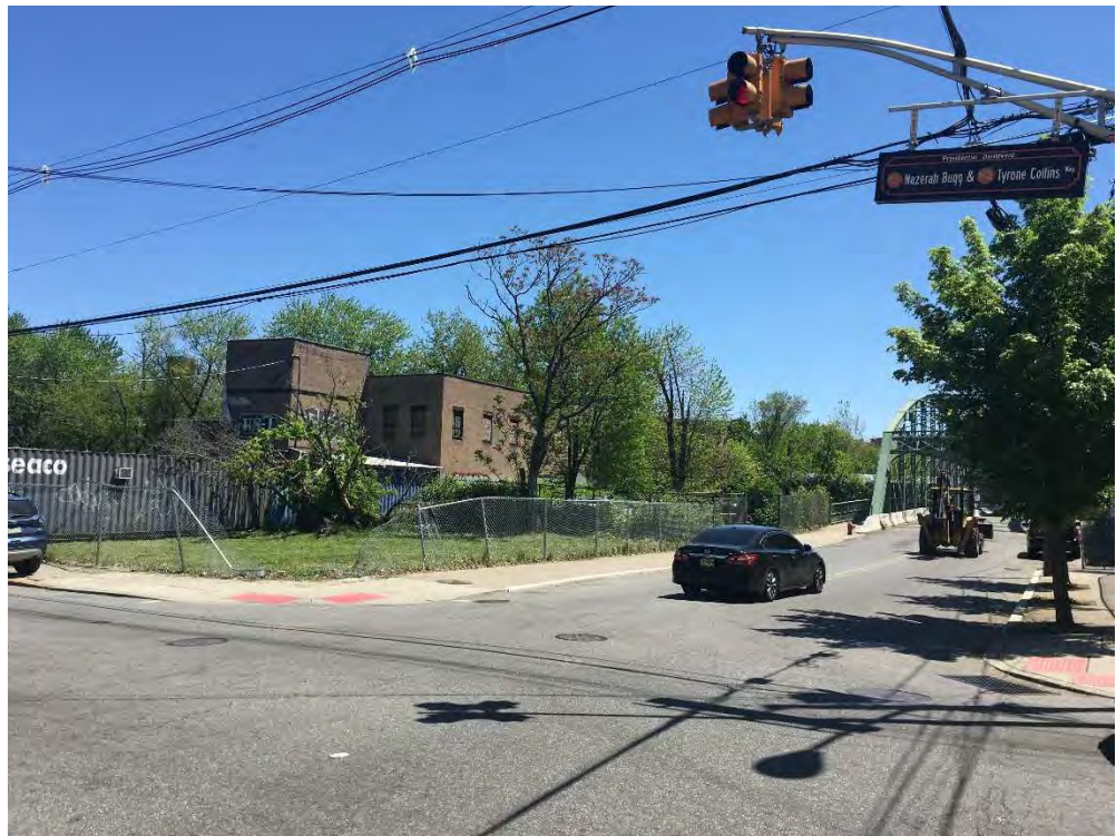
Abandoned property at entry to Arch Street Bridge
