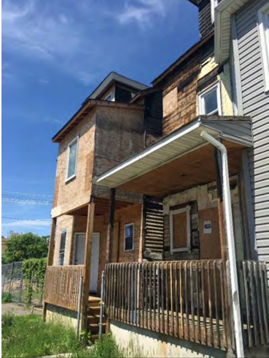
Vacant Property on N. Main St.
