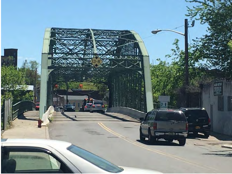
Entry to Arch Street Bridge
