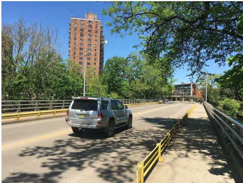
Main Street Bridge, looking toward the Northside
